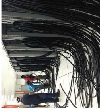
Supplied shielded control cables in Singapore 230KV sub-station.
